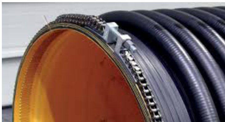
The external chain tensioner is tightened to a specific prescribed torque wrench setting against the internal spigot
